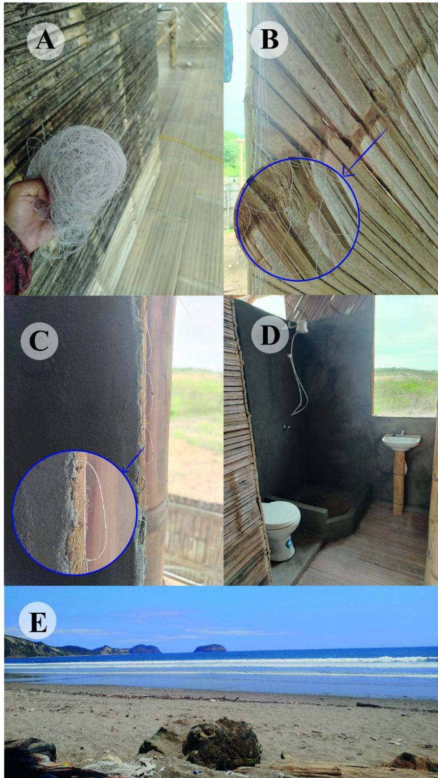
Fig 2. Reuse of damaged nylon fishing nets as reinforcement material in bamboo-based construction in Puerto Cayo, Ecuador. (A) Discarded and damaged nylon fishing net fragments prior to reuse. (B) Installation of the nylon net fixed to the bamboo wall structure before plastering. (C) Cement-plastered wall with portions of the nylon net visible along window edges, evidencing its incorporation as internal reinforcement. (D) Final plastered surface after completion of construction. (E) Panoramic view of Puerto Cayo beach, illustrating the coastal context where artisanal fishing activities and construction practices coexist. Source: Photographs by Hernán Orellana-Vásquez.
